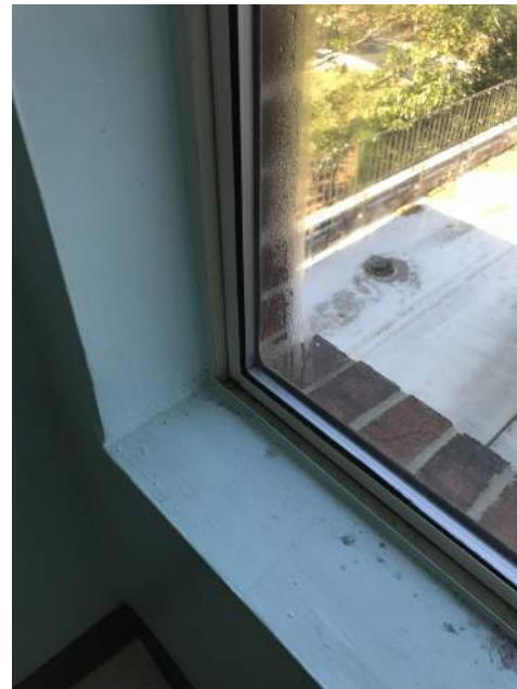
Existing windows showing condensation
