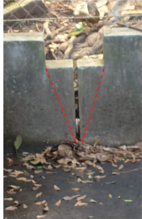
Image: this photograph displays the existing weir construction and the proposed cut lines to widen the notch while retaining its stormwater detention function.
